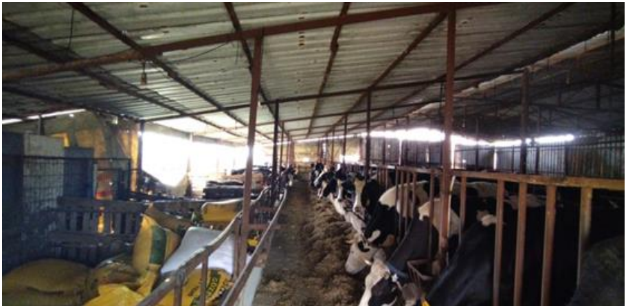
Figure 4. An example of a shelter roof covering
