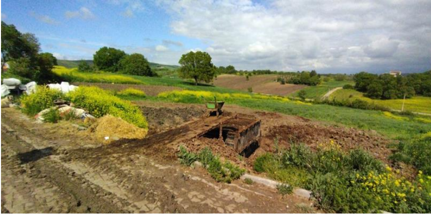
Figure 6. An example from the outdoor manure storage area
